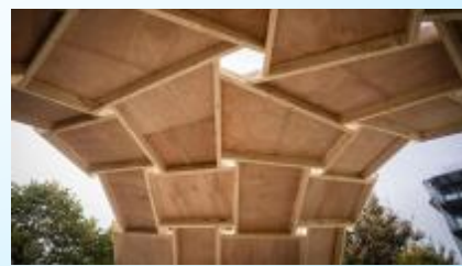
A shell nexoade structure braced with planar panels
