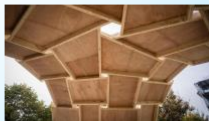
A shell structure braced with planar panels
