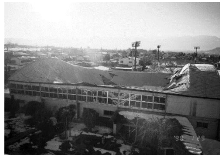
Figure 1 Gymnasiums collapsed under the unexpected heavy snow
